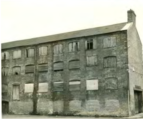
Abandoned flannel flannel mill
